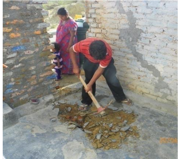
Digging a pit for installing in the courtyard.
