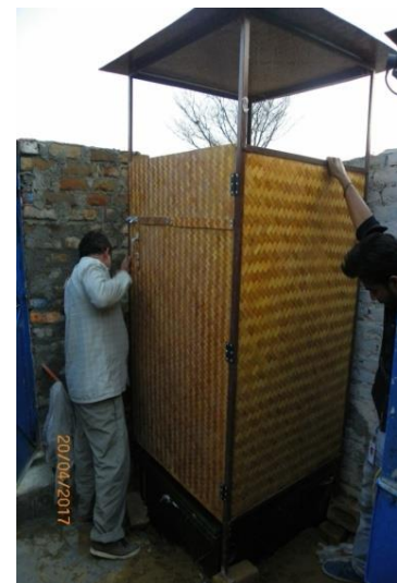
Fixing the cubicle
