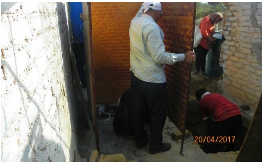
Assembly of cubicle panels
