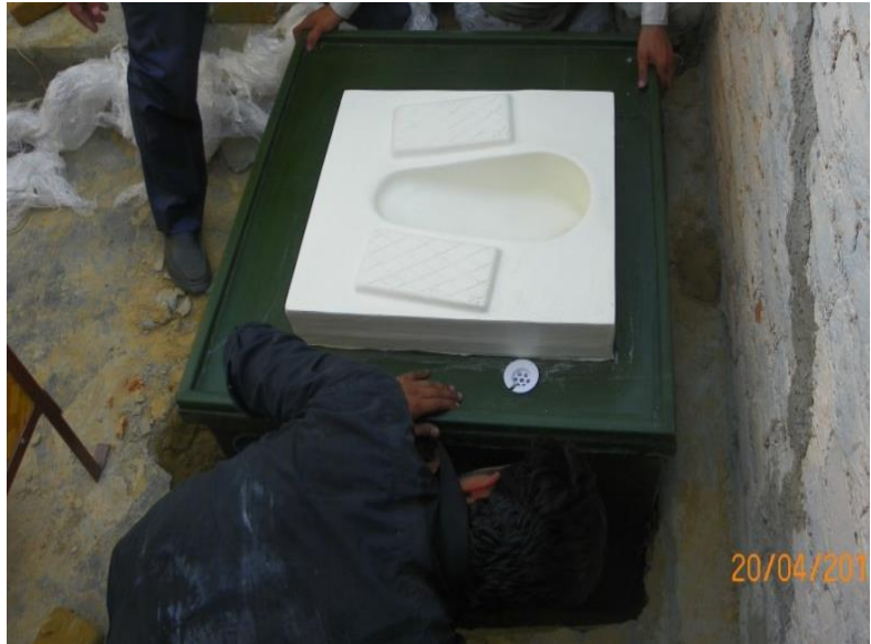
Fixing seat on the Bio Digester
