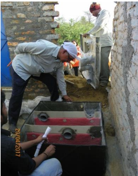
Installing the Bio Digester
